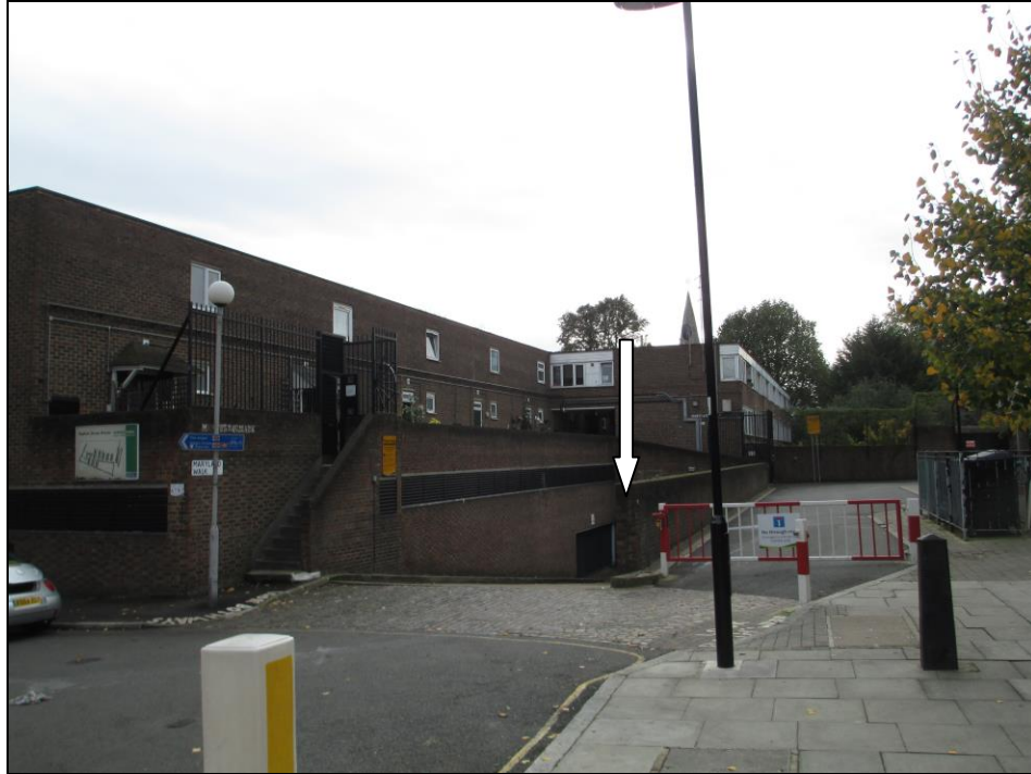
View from Popham Street looking towards the entrance to the site
